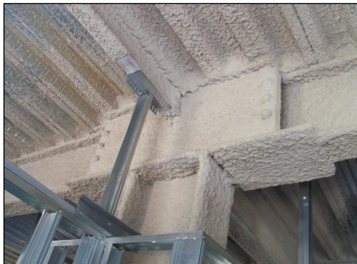
Figure 2 – Photograph of a Sideplate system. This is a moment frame that connects columns to beams and girders and can be single or double sided, shown above is a double-sided connection. Spray-on fireproofing has already been applied to the structural steel at this point of construction. Personal photograph taken by Chris Pozza.
