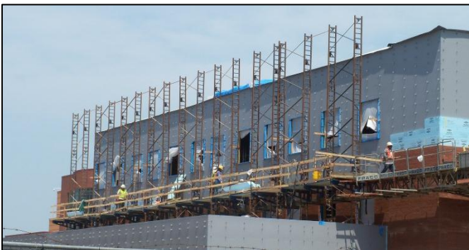
Figure 9 - View looking at southwest elevation. A MasonKing lift is required in areas where work is done above rooftops. These lifts have to be simultaneously cranked by hand to be lowered or raised. Personal photograph taken by Chris Pozza.
