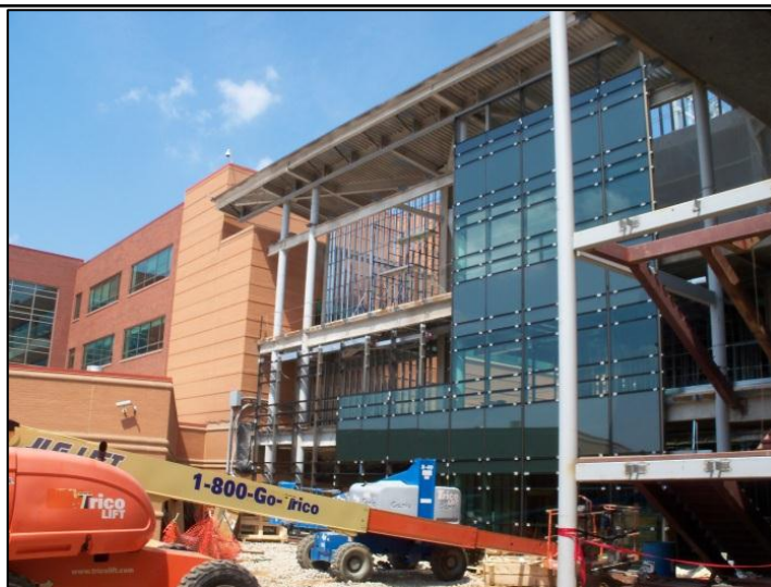
Figure 11 - View of west elevation curtain wall system under construction. The boom lift used during construction of the façade system can be seen at the bottom of the photo. Personal photograph taken by Chris Pozza.
