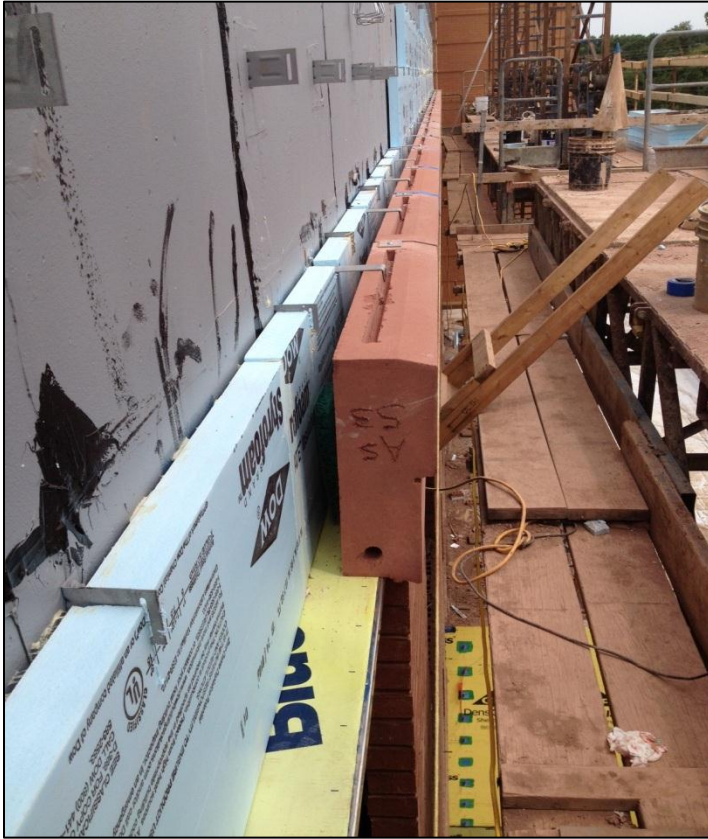
Figure 6 - Precast concrete can be seen above which make up the accent band along with east elevation. Personal photograph taken by Chris Pozza.
