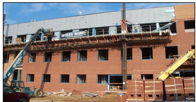
Figure 10 - View looking at east elevation. Fraco Lifts are used around exterior to provide efficient flow of construction along a large percentage of elevation at a time. Materials are lifted into place with a boom lift. Personal photograph taken by Chris Pozza.
